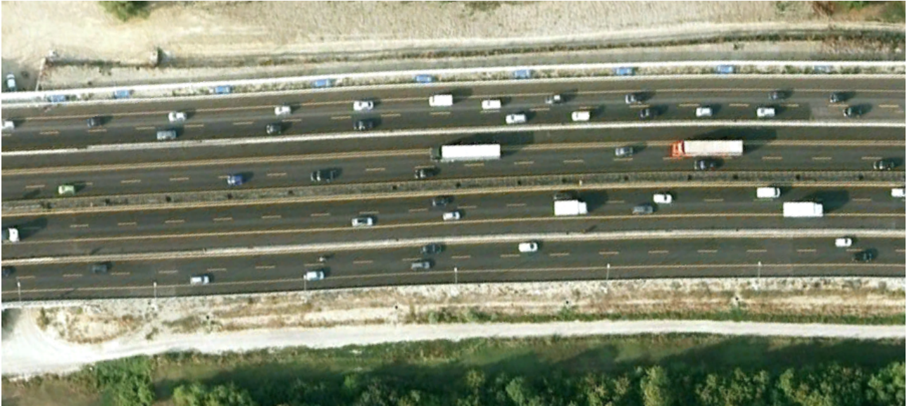
Figure 1. Aerial view of A14 north of Bologna, showing “inner” (transit) motorway and “outer” (local) motorway
