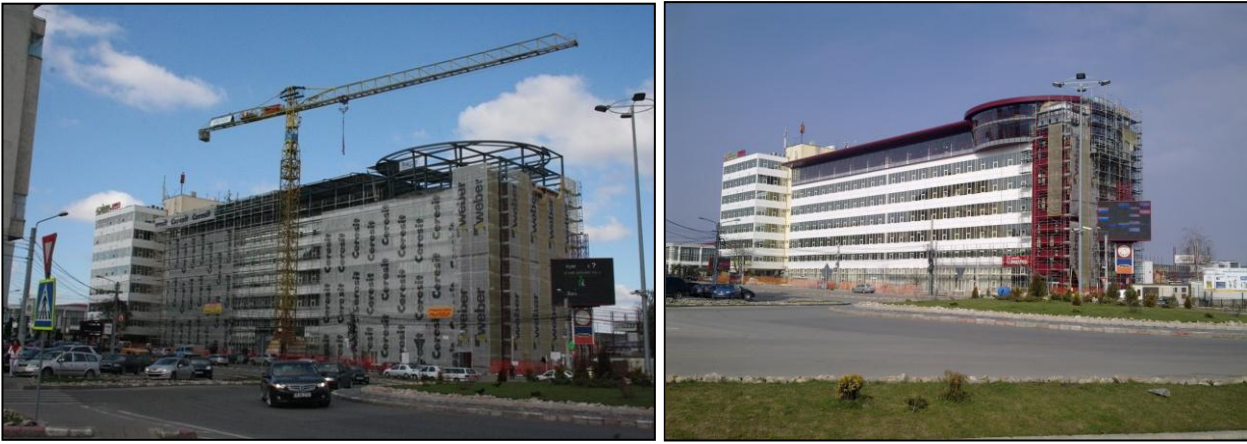
Figure 7. Intermediate and actual stage of the building.
