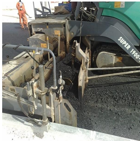
Figure 8. Asphalt laying
