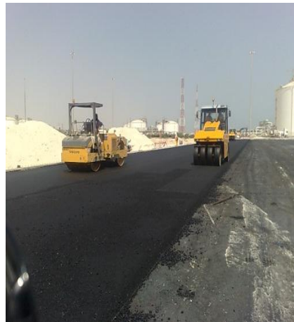
Figure 9. Bituminous layer compaction
