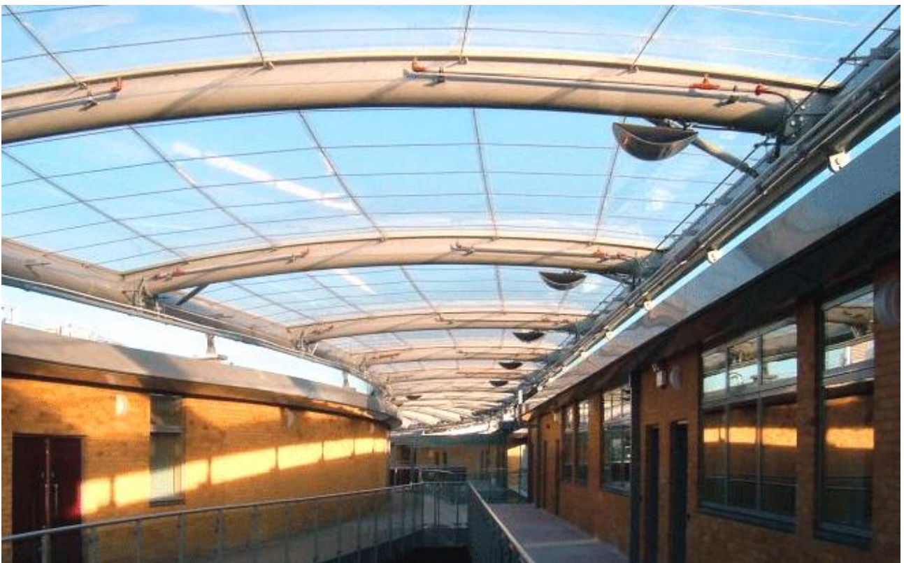
Figure 4. School in Lancashire, Great Britain (2008)
