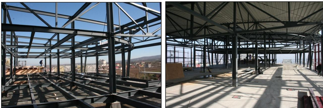
Figure 6. Structure during erection.
