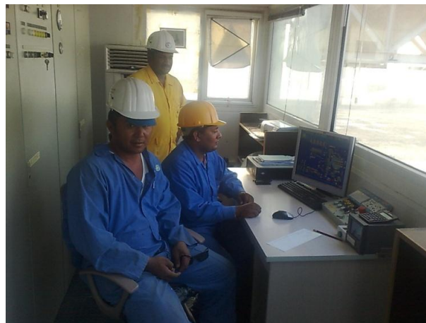
Figure 2. Asphalt plant control room
