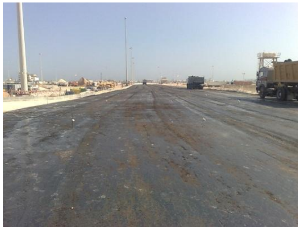
Figure 7. Priming with MC70
