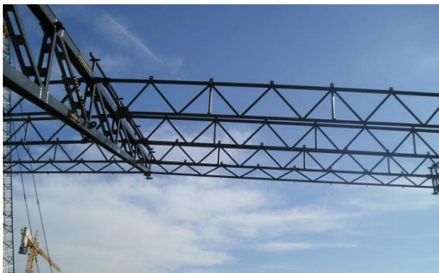
Figure 9. The longitudinal trusses
