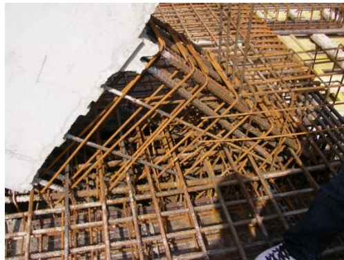
Figure 12. The monolithization of the joints of the inclined stepped beam
