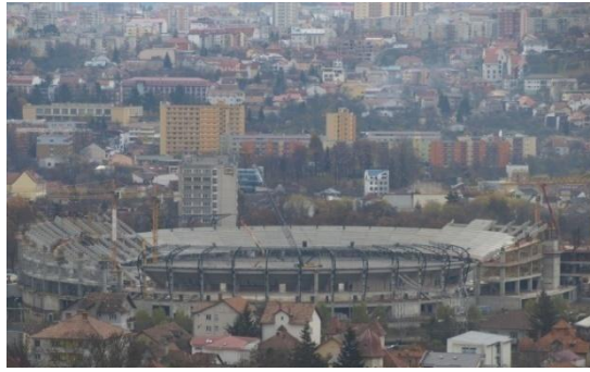
Figure 2. The stadium is under construction
