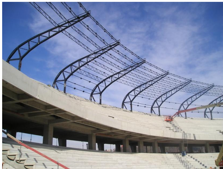
Figure 5. The steel structure of the roof: under construction.
