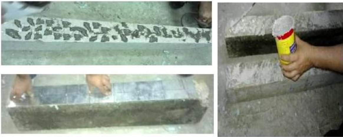
Fig. 7. Fixing the steel plate strengthening layer.
