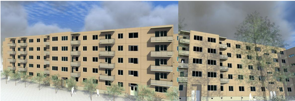
Figure 5. Case study building.
