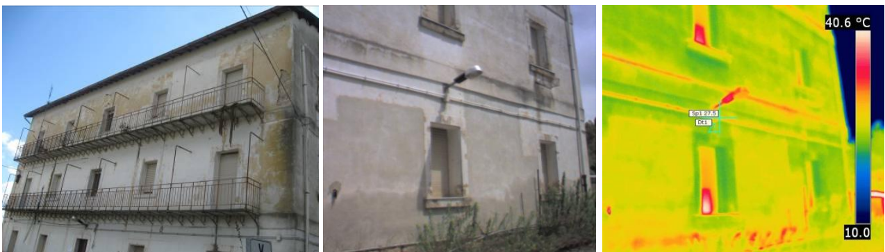
Figure 15. Dorms in Enna and their brick-bans masonry showed in thermography
