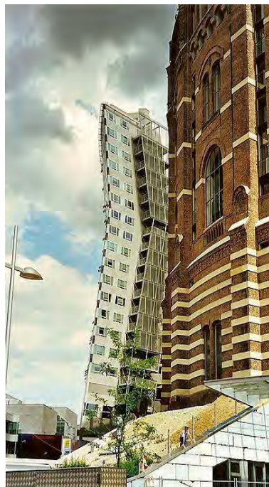
Figure 2. Gasometer B – exterior view
