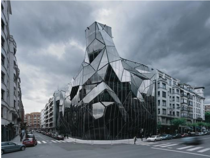
Fig. 3 BHD Exterior view (photo www.archdaily.com - Aleix Bague)
