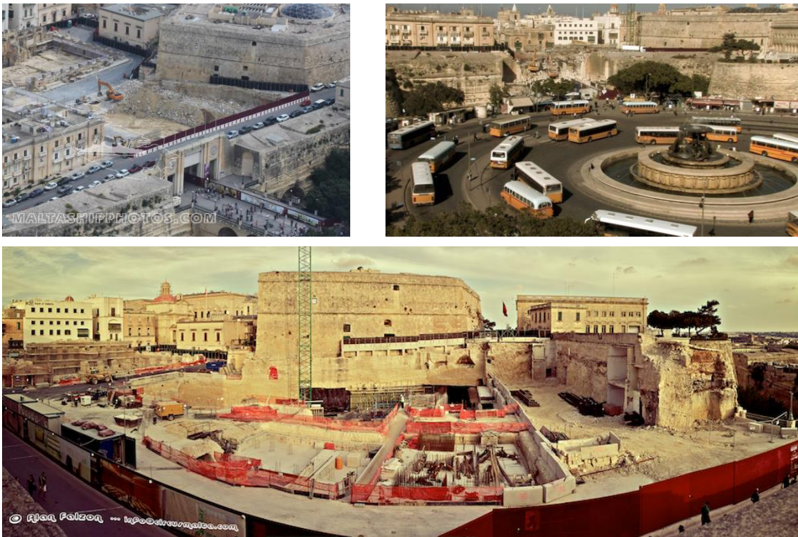
Fig. 38-40 Pictures showing the development of the demolition of the fourth gate
