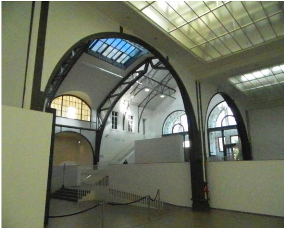
Figure 6. Central hall - the original structure was kept
