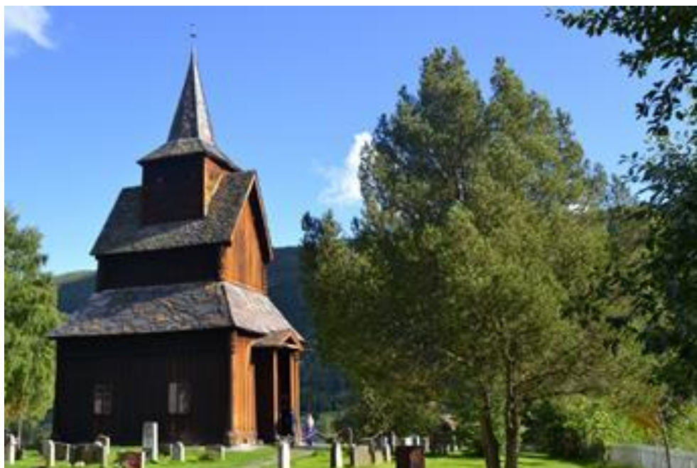
Figure 11. Torpo Church, Hallingdal, Norway
