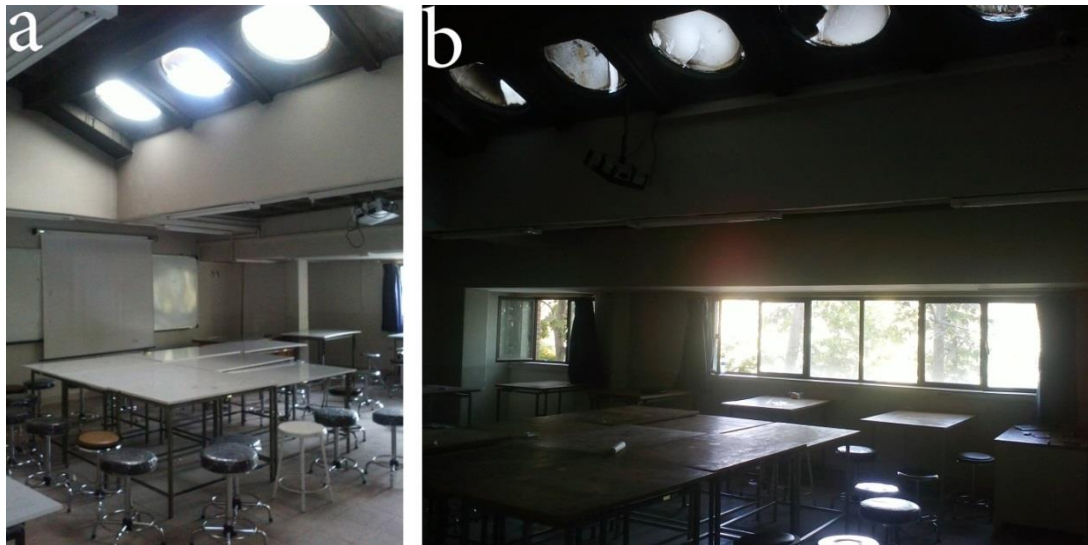
Figure 6: Ceiling skylights in the first floor ateliers (photos by the authors) (a) Related to optimal performance of ceiling skylights in one of the north-facing ateliers on the first floor with clean and healthy skylights (b) Related to poor performance of ceiling skylights in one of north-facing ateliers on the first floor with dirty and damaged skylights.
