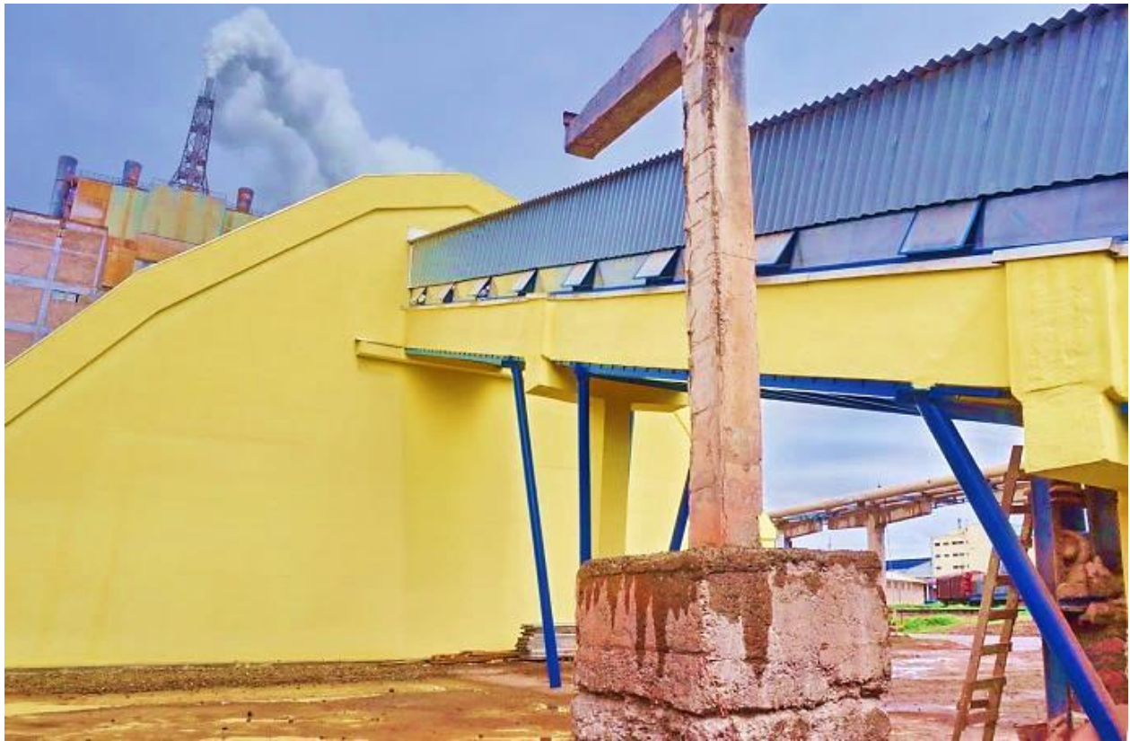
Photo 14. Post rehabilitation trestle
