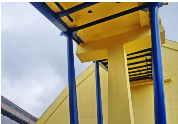
Photo 15. View of the rehabilitated trestle in the pillar area
