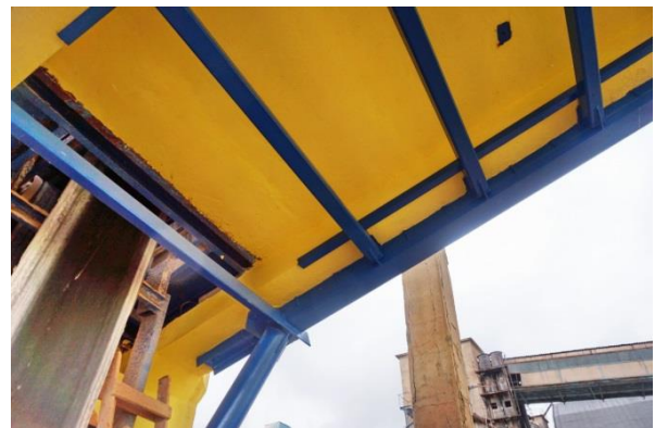
Photo 16. View of the rehabilitate trestle near the conveyor belt stretcher
