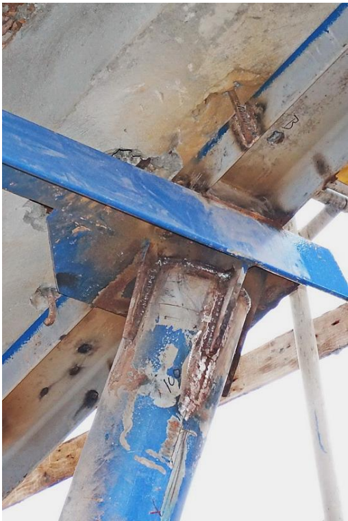
Photo 5. The same as in Fig. 7, execution
