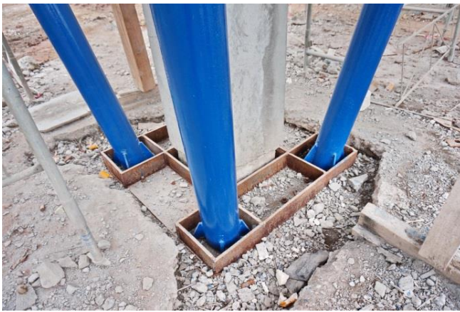
Photo 8. Execution of the system to support trestle on the foundation
