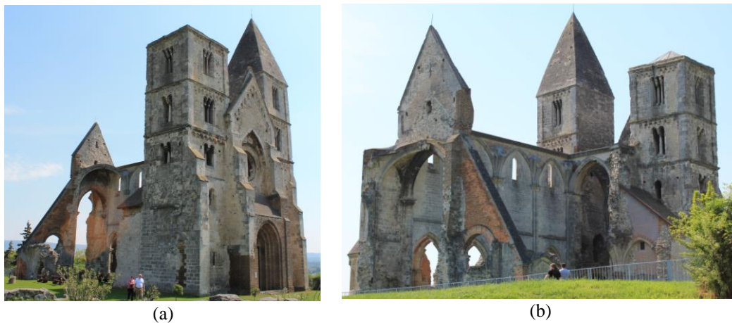
Figure 1. Zsámbék church: (a) western and (b) northern views (09/06/2014).
