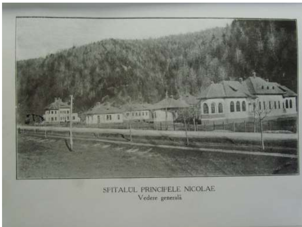
Figure 5. Prince Nicolas Hospital – general view – historical image.[5]
