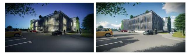
Figure 3. Night render / Day East elevation render: both image include vertical sun shading system from East sides of the building with the water waves form (4)
