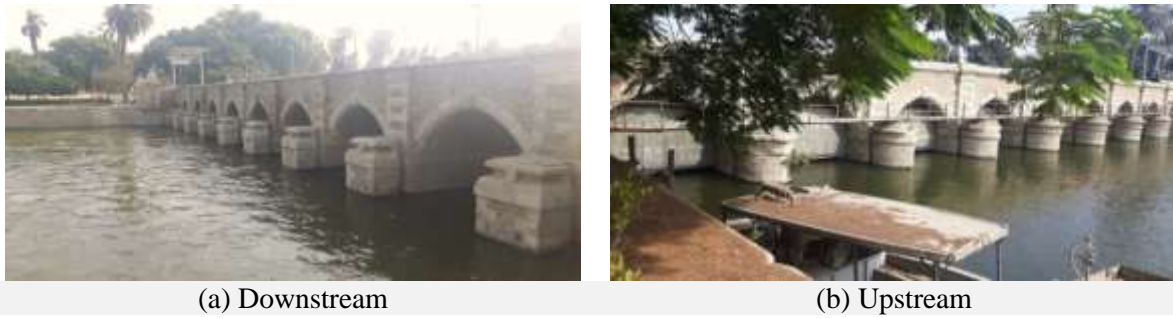
Fig.1 The downstream and upstream of the barrage
