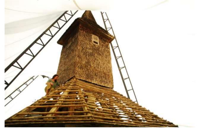
Figure 1. View of the open roof framing in Crivina de Sus.
