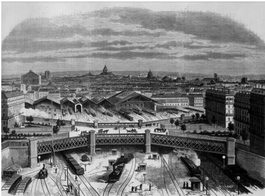
Figure 3. Auguste Lamy, Paris. Bridge Erected on the Place de l’Europe, over the Western Region Railway . Published in L’illustration , 11.04.1868.
