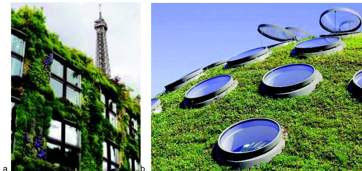
Fig. 2.2 – a. Musée du quai Branly, Paris, arh. Jean Nouvel; b. California Academy of Science, San Francisco, arh. Renzo Piano [78;102]
