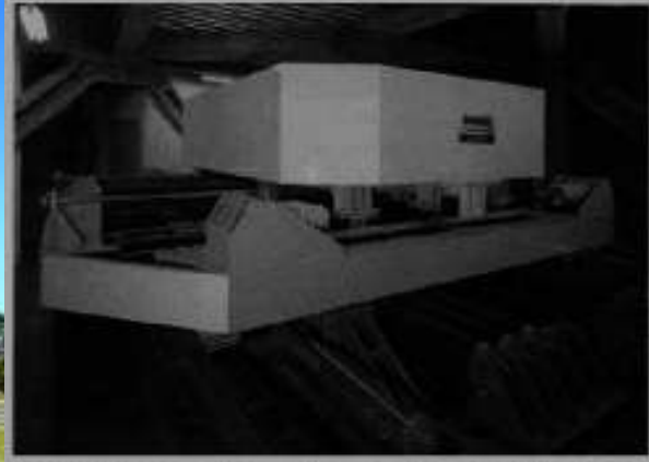
Fig. 1.4.5 Chiba Port Tower tuned mass damper [126]
