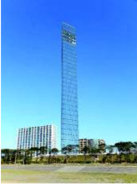
Fig. 1.4.4 Chiba Port Tower [125]
