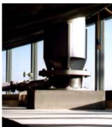
B- izolator cauciuc laminat
