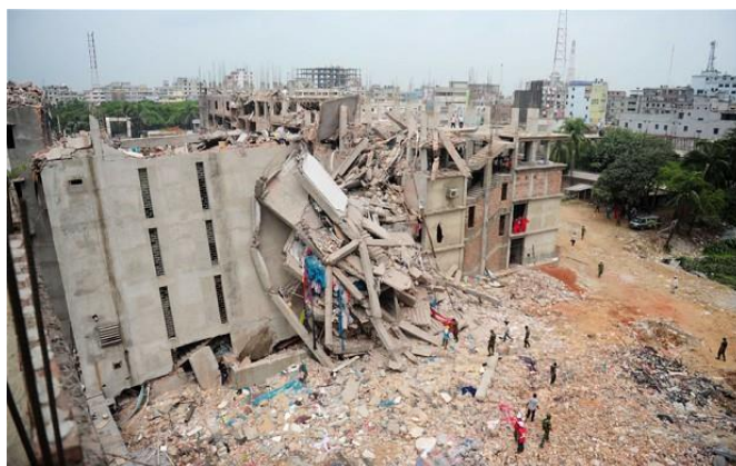
Figura 1.6 Colapsul clădirii Rana Plaza (Bangladesh, 2013) [12]
