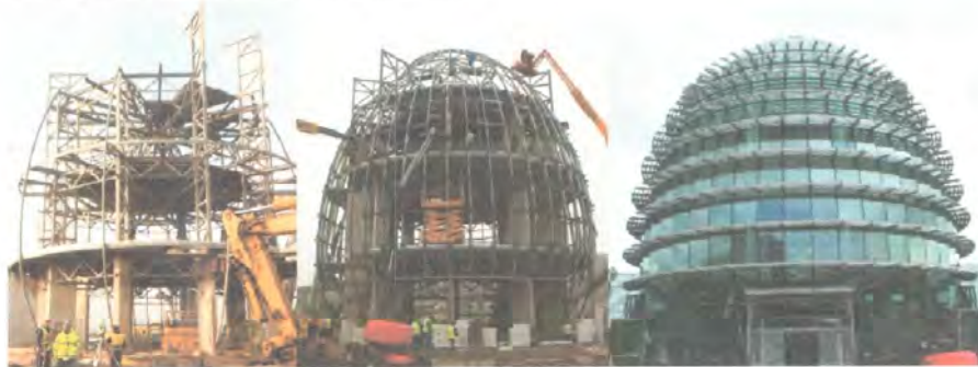
Fig. 12 Erection phases of C1
