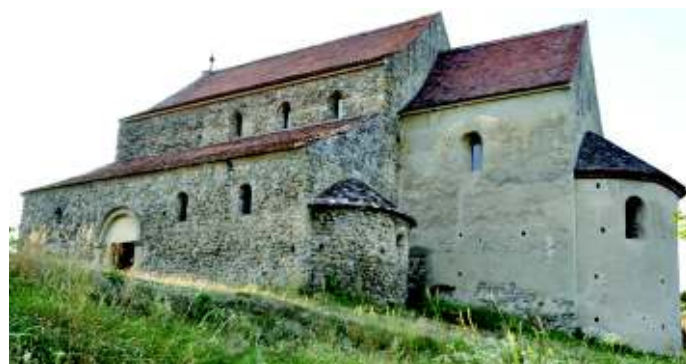
b. south façade
