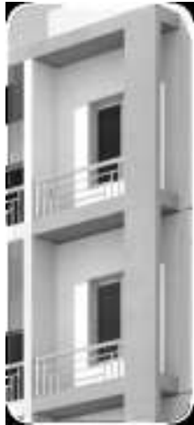
a. the sunshade used on the south façade
