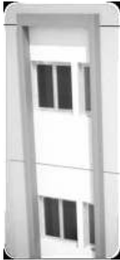
b. the sunshade used on the east and west façades
